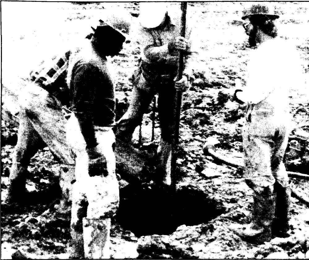
Make a hole, make it wide: Construction workers prepare one of the foundations for support columns of the new library/academic complex .
