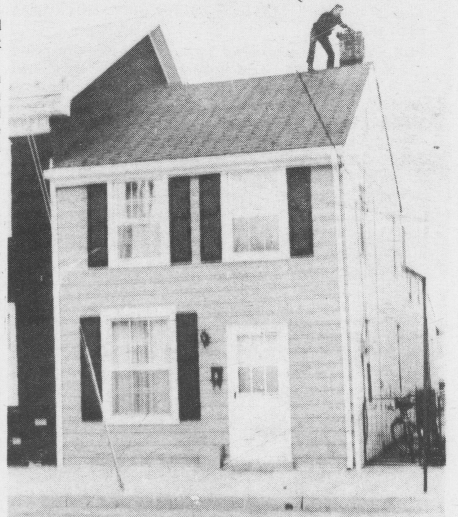
Jim working on the roof
