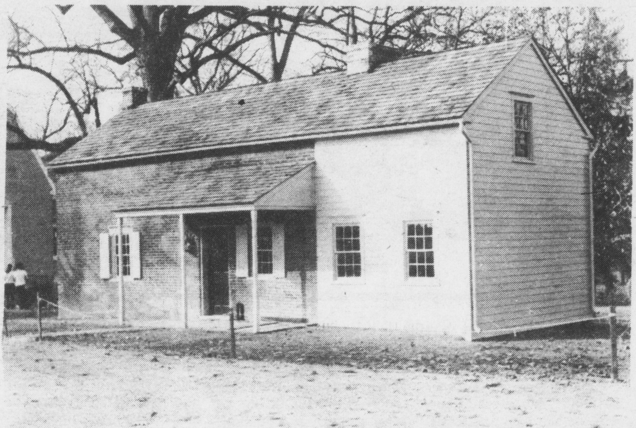
The study house of Donegal Presbyterian Church, recently restored under the direction of Jerry Martin of Marietta. The study house was originally built in 1810.
