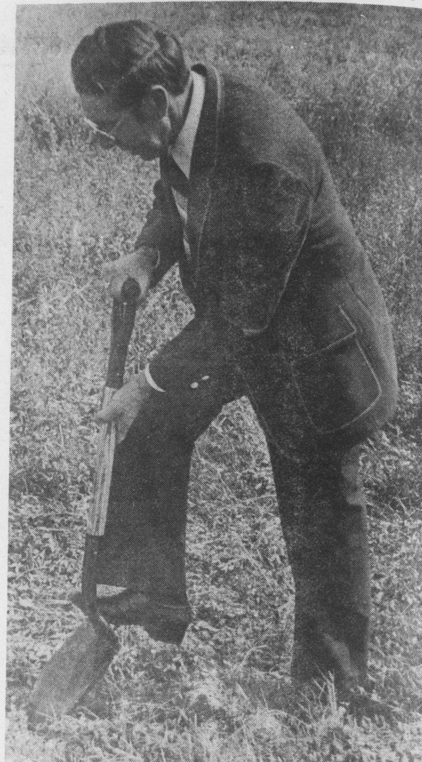
Rev. Leroy Hoover breaks ground for the new church.
