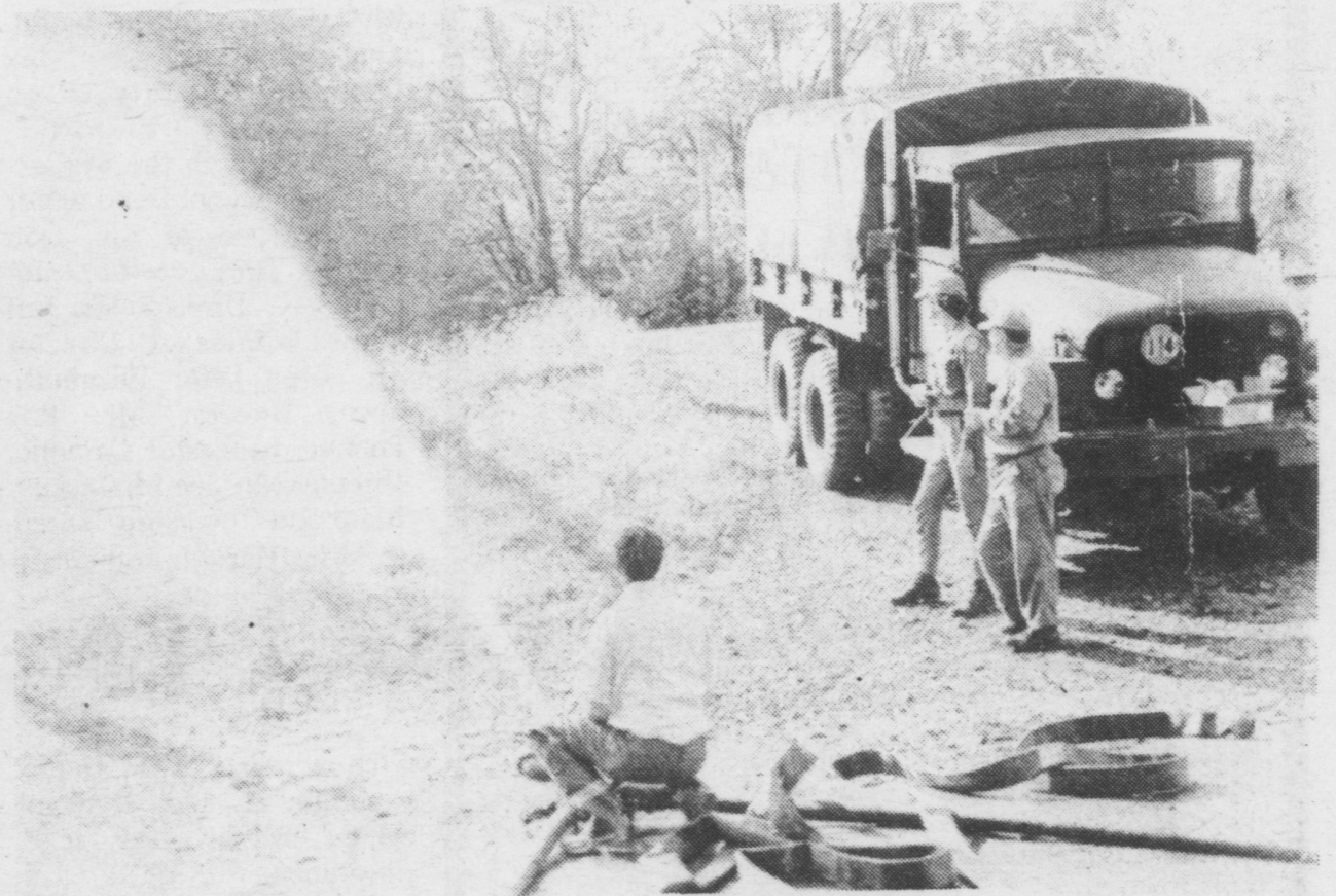
Firemen pumping out basement on Front Street
