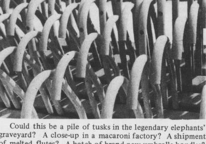
graveyard? A close-up in a macaroni factory? A shipment of melted flutes? A batch of brand-new umbrella handles? Actually, they're stacked-up supports for electric wires in a \$4,900,000 set of dust collectors being installed by Pennsylvania Power & Light Company to clean flue gases at its Sunbury Steam Electric Station in Shamokin Dam, Pa.
