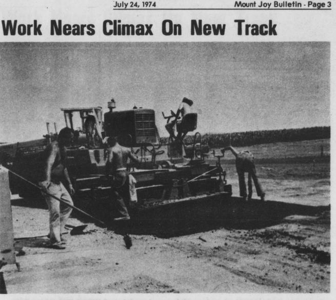
WORKMEN PUT DOWN first of three layers of the surface for Donegal high school's new \$100,000 running track, located immediately north of the present baseball field. Final surfacing — a special, resilient material — may be laid later this week.
