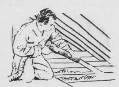
Are you sure you have enough insulation?— Adequate insulation in your home can reduce heating costs by as much as one-third. Even in homes thought adequately insulated a few years ago, some additional insulation, particularly in the ceiling, may produce substantial savings. And, as shown below, it's an investment that pays for itself quickly.
