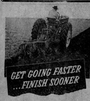
WITH THE JOHN DEERE 3-POINT HITCH for "50," "60," and "70" Tractors, you hook up or change implements in far less time-get to work quicker-transport at faster speedshave greater maneuverability in close-quarter work. This 3-point hitch gives you a flexible, free-trailing implement with a minimum of side-draft-you save fuel, do more uniform work.
