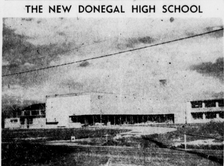
This view of the partially completed school shows the main entrance; the auditorium and gymnasium to the left and classrooms on the right.
