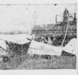
For the first time, liquid nitrogen fertilizer was transferred direct from a railroad tank car to a waiting plane. The plane flew 20 miles to a 1000-acre wheat field, sprayed its load, and returned to the siding for a quick refill-all in about 15 min-
