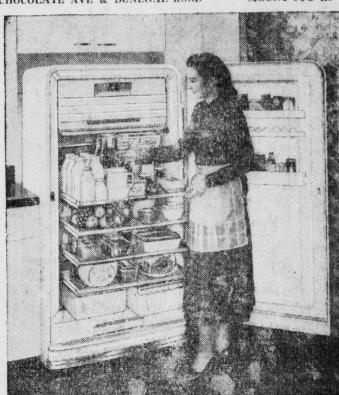
New Cycla-matic Frigidaire food freezer and refrigerator combination, just introduced, features shelves that glide out on nylon rollers for easy access, handy storage space on door, and a new kind of safe, constant cold called Levelcold. Upper compartment is zero-zone food freezer, completely insulated and sealed from rest of cabinet. Cycla-matic defrosting in refrigerator section automatically controls hu-midity and banishes frost before it collects.
