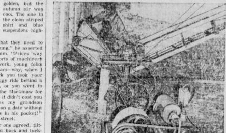
IT TOOK SOME DOING-but here's a wagon unloader rigged up to remove onions from wagon to elevator for transportation to storage building.
