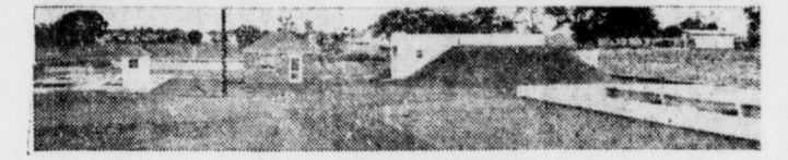
Sewage Treatment Works, Littlestown, Adams Co. Left, bar screen, primary and secondary tanks, re-circulating pump station. Center, control house. Right, Digester. Right foreground, Sludge beds. Rear left, filter.
