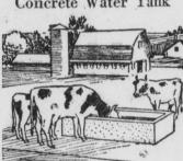
concrete livestock watering tank is watertight, furnishing an ample supply of fresh water in readily accessible troughs. A concrete pave-ment six feet wide around the tank is highly desirable to provide a clean, mud-free platform for livestock to stand on.
