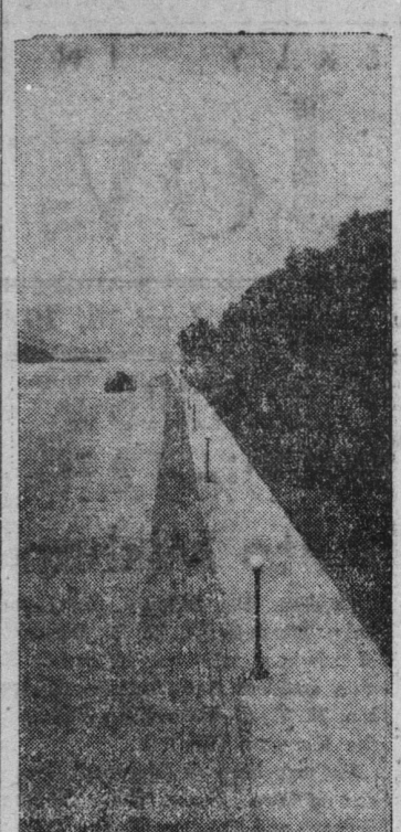
This concrete esplanade follows the river at Harrisburg for miles. It is a favorite promenade between beautiful River Park and the Susquehanna.
