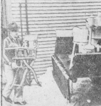
MINE CITY SINKS ... Residents of Shenandoah, Pa., shown evacuating homes as part of city built over anthracite mine caved in. Among relief offers to Burgess (Mayor) Andrew Barniak was first public activity of new Pennsylvania chain store council whose president, Scott Rea, pledged aid of chains in relief program. Cave-in was called worst in history of southern Pennsylvania region.
