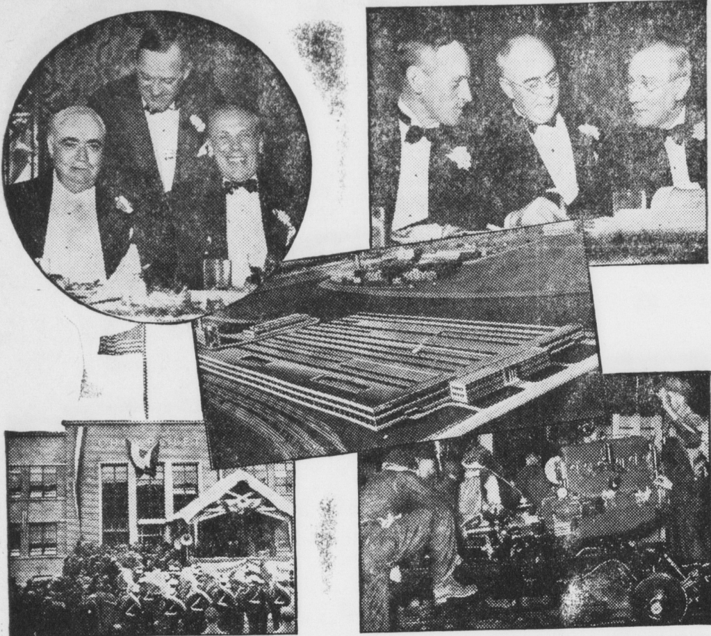
Governmental, state and civic officials joined with the principal executives of General Motors Corporation in the formal opening of the new 80,000-car-a-year Chevrolet assembly plant in Baltimore recently. The new plant (center) was dedicated with impressive ceremonies (lower left), and Chevrolet, Fisher Body and General Motors officials were guests of the Baltimore Association of Commerce at a formal banquet in the evening. W. E. Holler, vice-president and general manager of Chevrolet, is shown (standing) with Maryland's Governor, H. W. Nice, and Alfred P. Sloan, Jr., president of General Motors (upper left). M. E. Coyle, president and general manager of Chevrolet, is pictured in the upper right photo with Senator Millard Tydings (left) and Mayor H. W. Jackson, of Baltimore (right). Lower right shows the first motor car built in that city.
