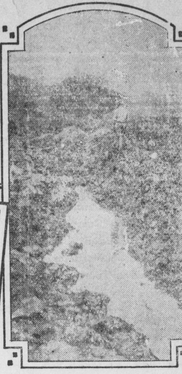
Draining a marsh begins in but a few minutes after the explosive has blasted the ditch.
