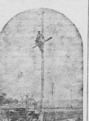
finding and clearing his Bell Telephone repairman and his "flivver" are hard to beat. The repairman is protected by rubber coverings which are placed around high tension wires whenever ft is necessary for him to climb through them
