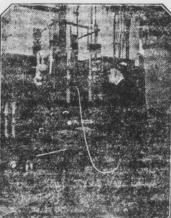
Pumping out the gas to make vacuum tubes in the Western Electric Company Laboratories. The complicated apparatus is needed to help prepare the tubes that make practicable long distance telephone and radio com-
