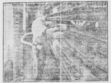
House cleaning in a Bell Telephone central office! Specially constructed vacuum cleaners with brush attachments are used for removing the dust from the thousands of telephone wires that terminate in the switchhoard.
