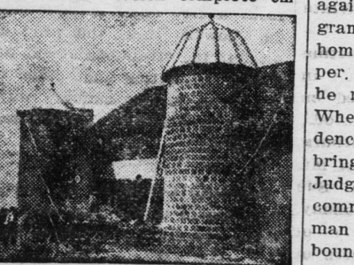
Oil Engine Filling Silo
