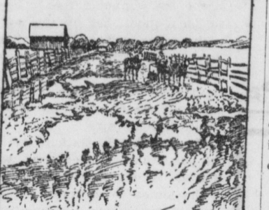
TYPICAL CLAY ROAD BEFORE IMPROVEMENT.
