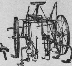
ment than will be done by hand hoeing or any cultivator made. This is simple and easily operated, and easily attached and detatched and invaluable grower of tobacco.
