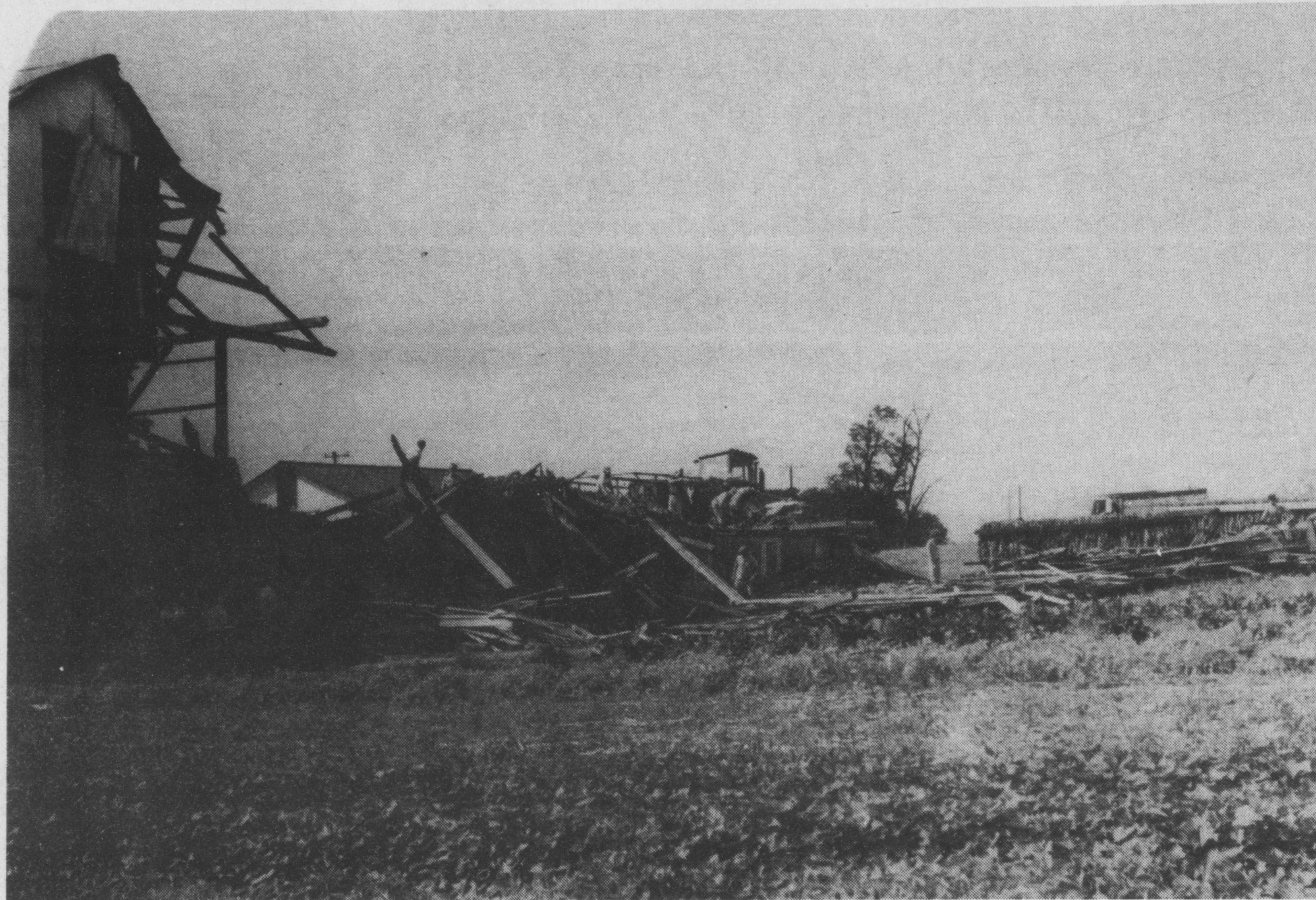
High, localized winds did damage to several barns and smaller buildings outside of Maytown Sunday night. Shown above are the remains of a large structure located at Colebrook and Rock Point Roads. Workmen were already clearing away the debris Monday morning.
