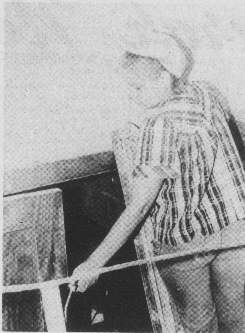
Painter works on the interior of the Marietta Jaycees' Center.
