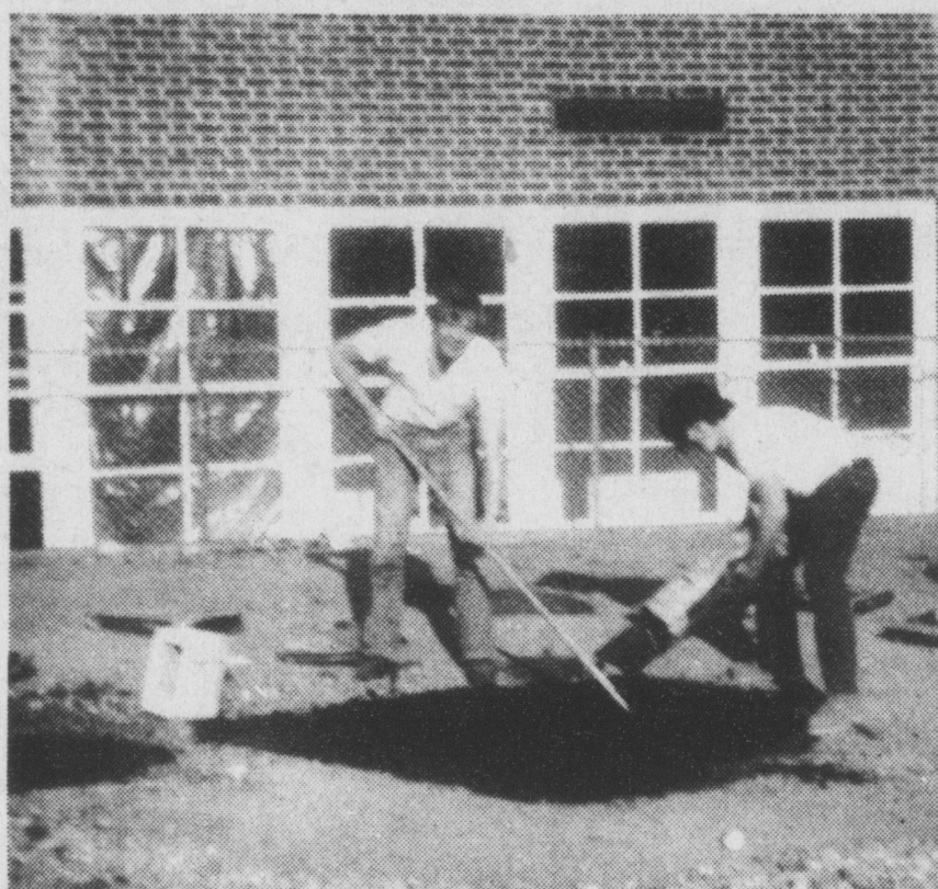
Gary Newton and Scott Neal fix holes behind the Jaycee building.
