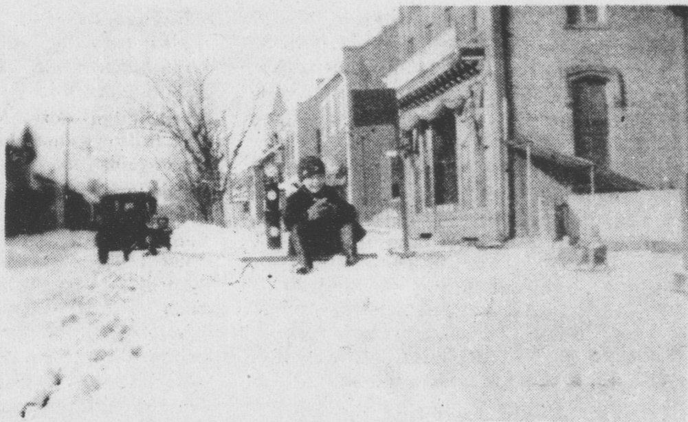
In this early photo of West Main Street, Mount Joy, George Brown III plays in the snow in front of what used to be Brown Brothers Hardware. Today J.B. Hostetter and Sons, Inc. makes its home in the same building. The photo was provided by Bruce Brown of Mount Joy.
