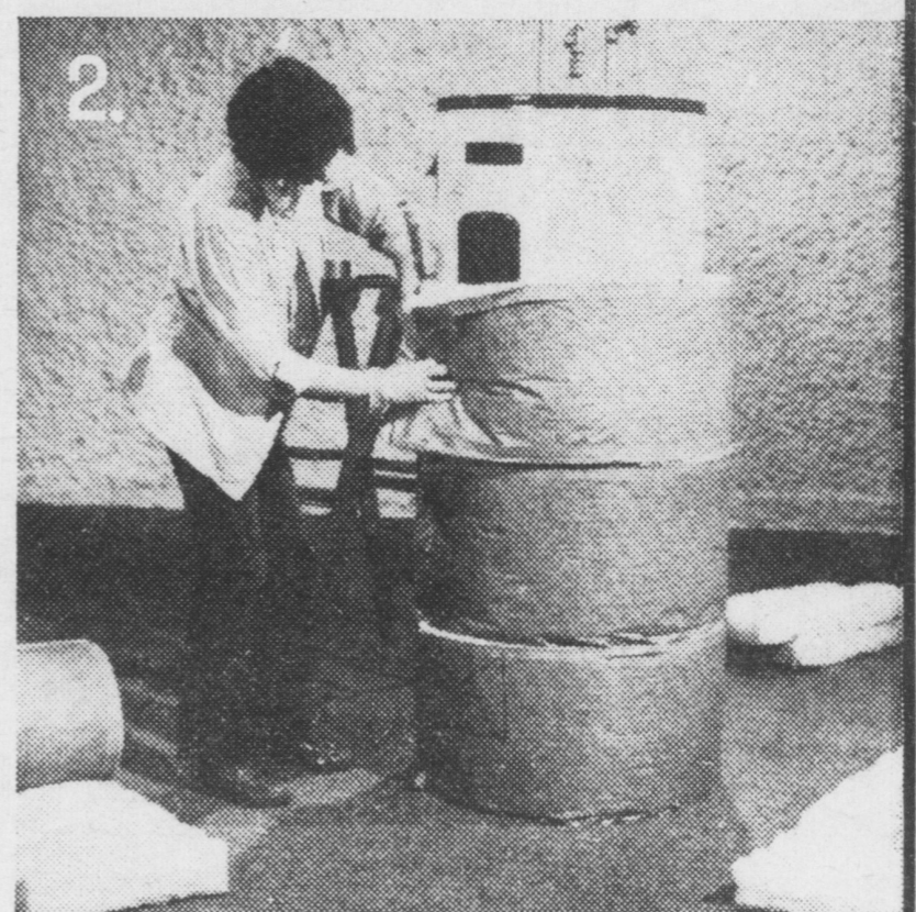
Cut strips of insulation to wrap around your tank . . . two half-circle pieces to cover the top (do not cover temperature-pressure relief valve). Mark thermostat locations and apply duct tape to all seams.
