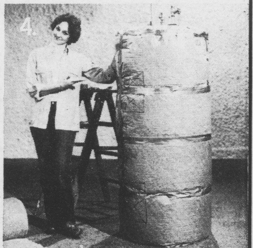
Granted . . . electric water heaters are factory insulated. But, when you can make yours a little more efficient simply by wrapping it in 3½ inches of ordinary household insulation . . . why not?
