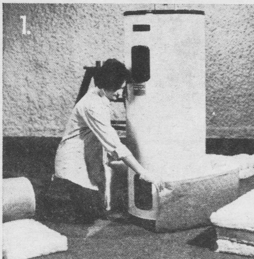
Adding a blanket of insulation to your electric water heater is quick and easy. Inexpensive, too. About 30 minutes of your time and about $10 worth of materials should do it.
