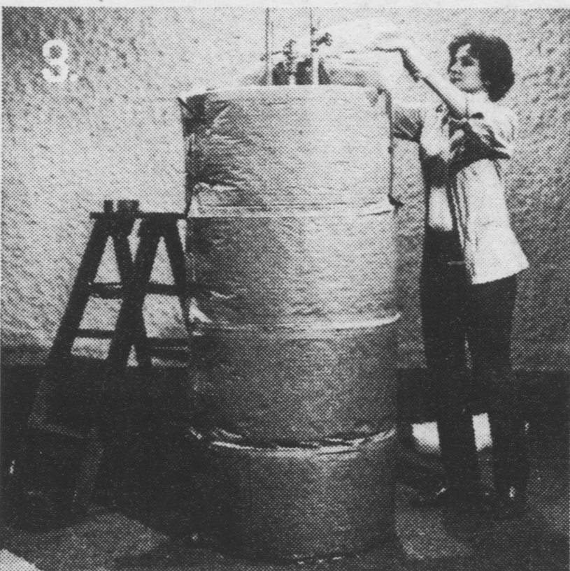
Because insulation helps contain heat in the tank, it saves energy and money. In less than six months your extra insulation can pay for itself. After that, savings continue for years!
