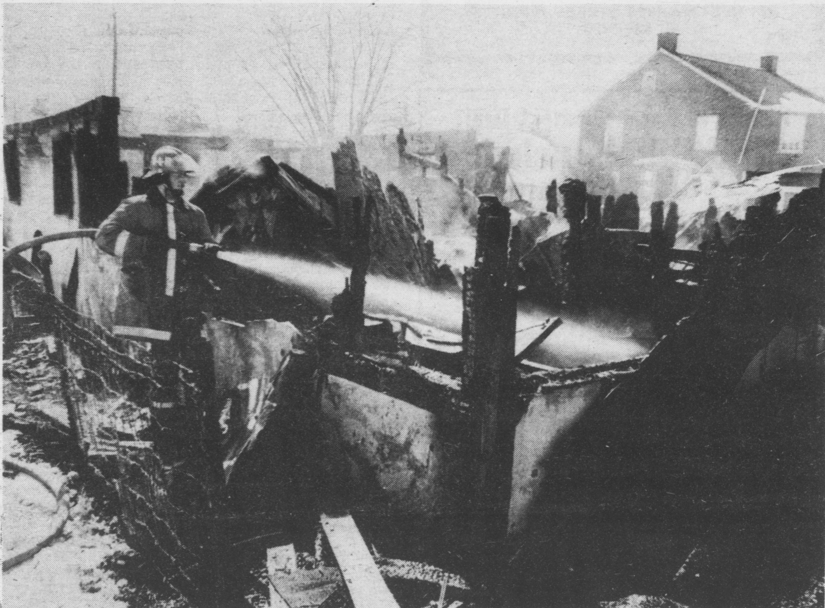
A fireman sprays water onto the smoldering ruins of Ellis's house.
