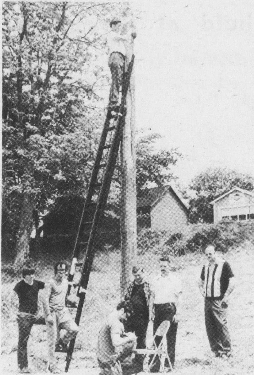
Photo shows some of the men of the Pioneer Fire Company stringing lights for the company's carnival this Saturday.
