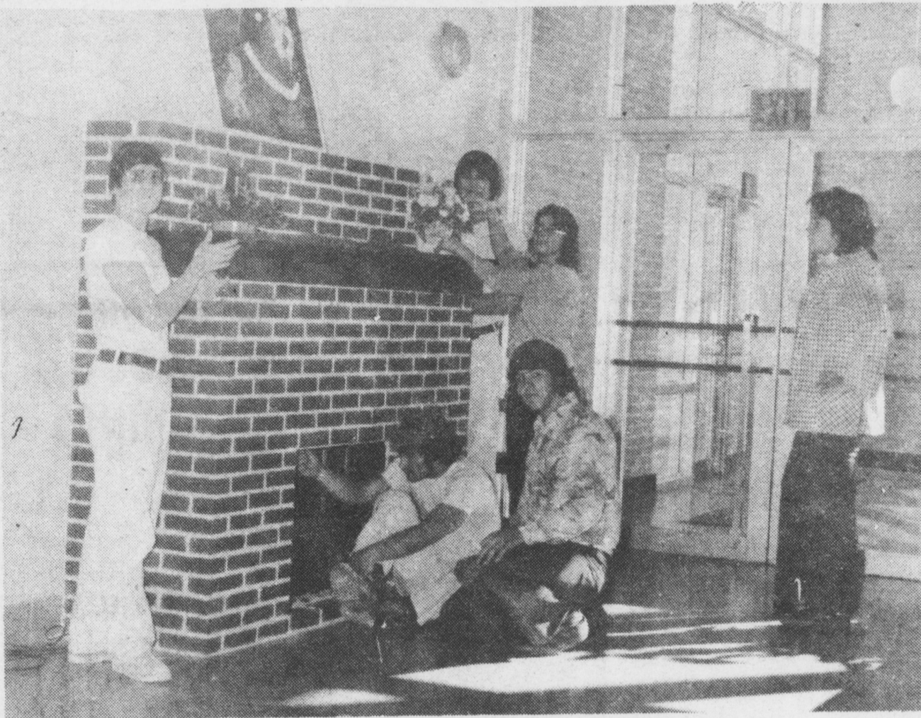
Rick and Brett Funk, Eugene Mellinger, Pontia Hossler, Renee Husband and Rick Gibble at work on the Vo-tech fireplace.
