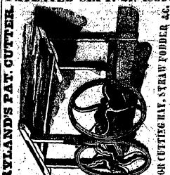
The merits of this Machine consist, in part, in the nttachment of curved knives to the arms of the cutting-wheel, the shearing our across the mouth-piece, the great power and directness of the blow, by which er than is required by any other Macaine; those combined with its durability and simplicity of carstruction, command public attention. Nothing heole to get out of order, but what a boy could remedy with a pocket wrench.
