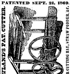
The merits of this Machine consist, in part, in the attachment of curved knives to the arms of the cutting-whoel, the shearing cut across the mouth-piece the great power and directness of the blow, by which treble the volume of material is cut, with less power than is required by any other Machine; those combined with its durability and simplicity of construction, command public aftertion. Nothing liable to get out of order, but what a boy could remedy
