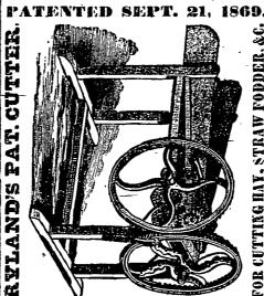
The merits of this Machine consist, in part, in the attachment of curved knives to the arms of the cutting wheel, the shearing cut across the mouth-piece, the great power and directness of the blow, by which trel le the volume of material is cut, with less power than is required by any other Machine; those combined with its durability and simplicity of construction, command public attention. Nothing liable to get out of order, but what a boy could remedy with a pocket wrench.
