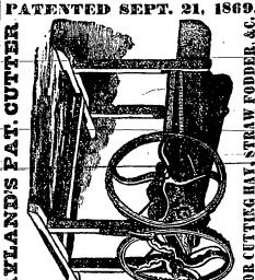
The merits of this Machine consist, in part, in the S P R I N C attachment of curved knives to the arms of the cut-ting-wheel, the shearing cut across the mouth-piece, the great power and directness of the blow, by which trelile the volume of material is cut, with less power than is required by any other Machine; those combined with its durability and simplicity of construction, command public attention. Nothing lia-ble to get out of order, but what a boy could remedy
