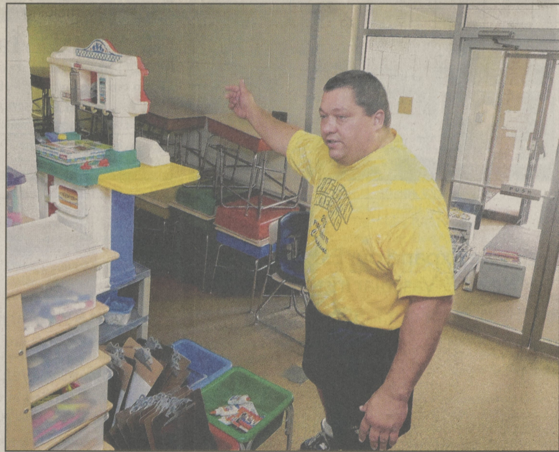
Lake-Lehman Superintendent James McGovern describes the renovations currently underway at Lehman-Jackson Elementary School to accommodate the district's new day care facility.
