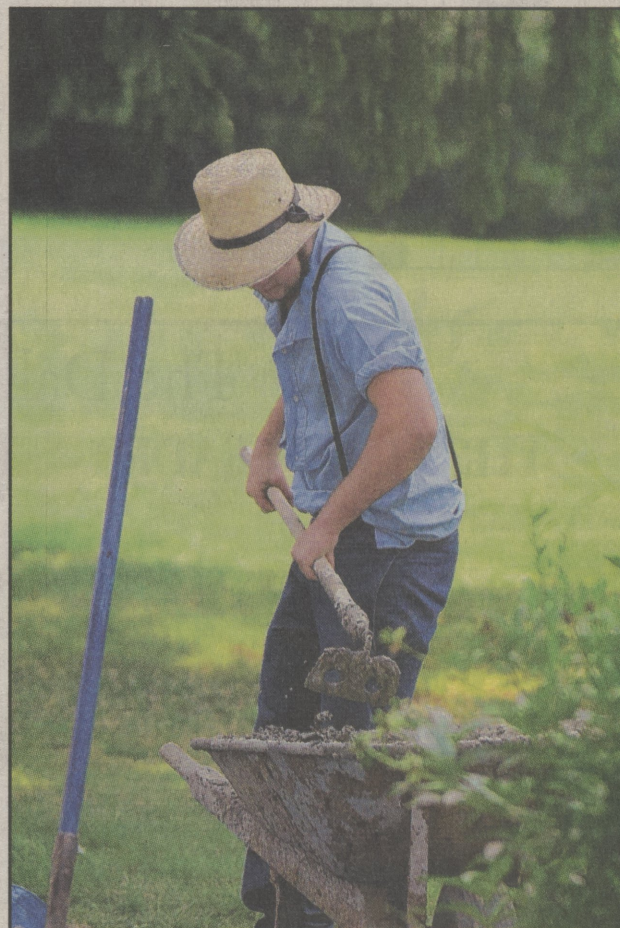
Leroy Mast Jr., an Old Order Amish from Warren Center, PA, his father and two brothers work to save the old church hall at the Methodist Church in Orange.
