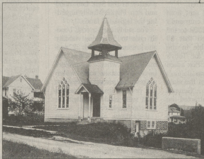
This postcard shows the old Shavertown United Methodist Church (1903 building). It stood in the same spot as the new one, on land given to the church by local farmer Theron Ferguson. The postcard was sent to the congregation by the minister, W.S. Wilcox.
