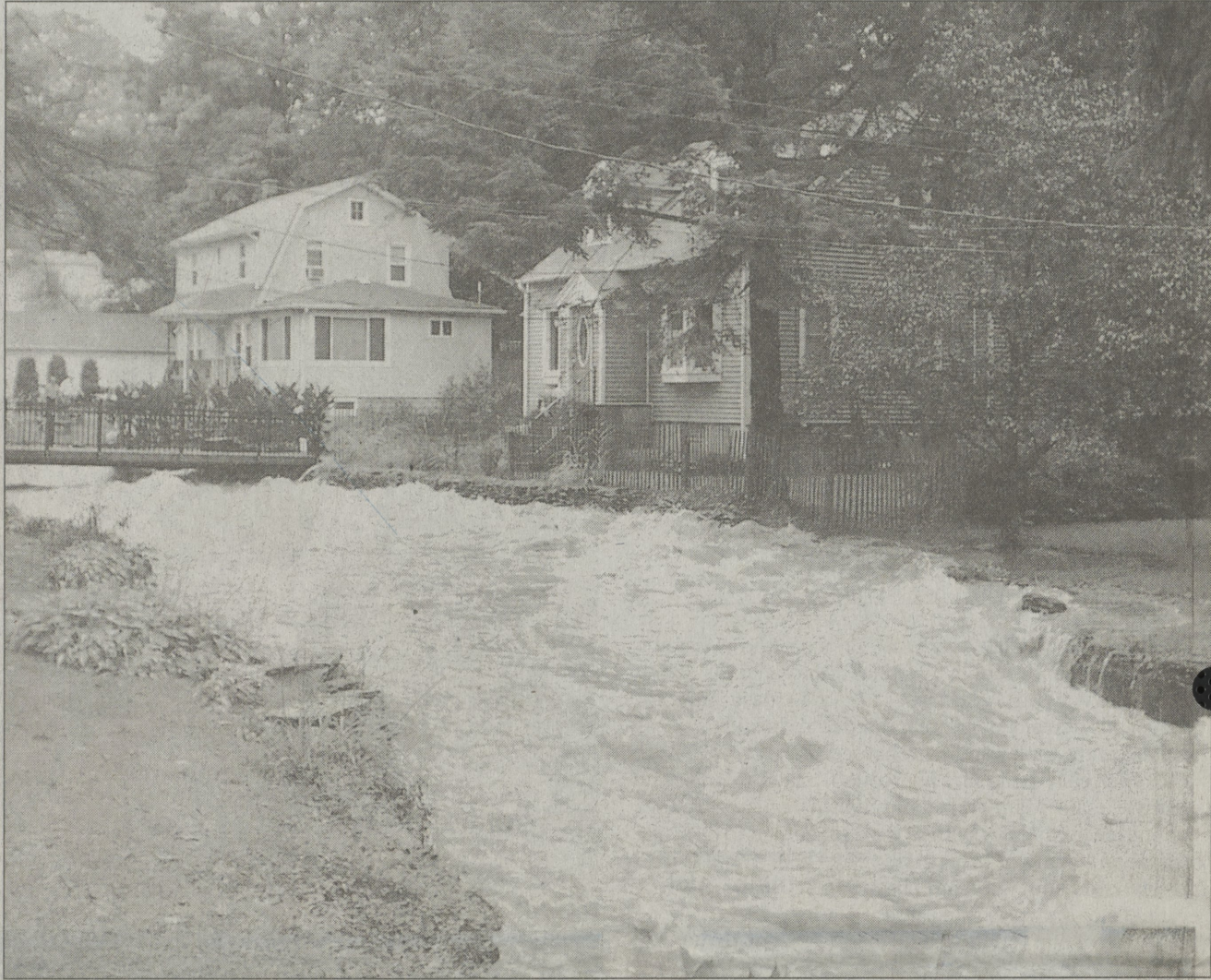
Toby's Creek smashed against a rock wall that protects homes just off Route 309 in Shavertown. Private bridges connect the properties to North Main Street.
