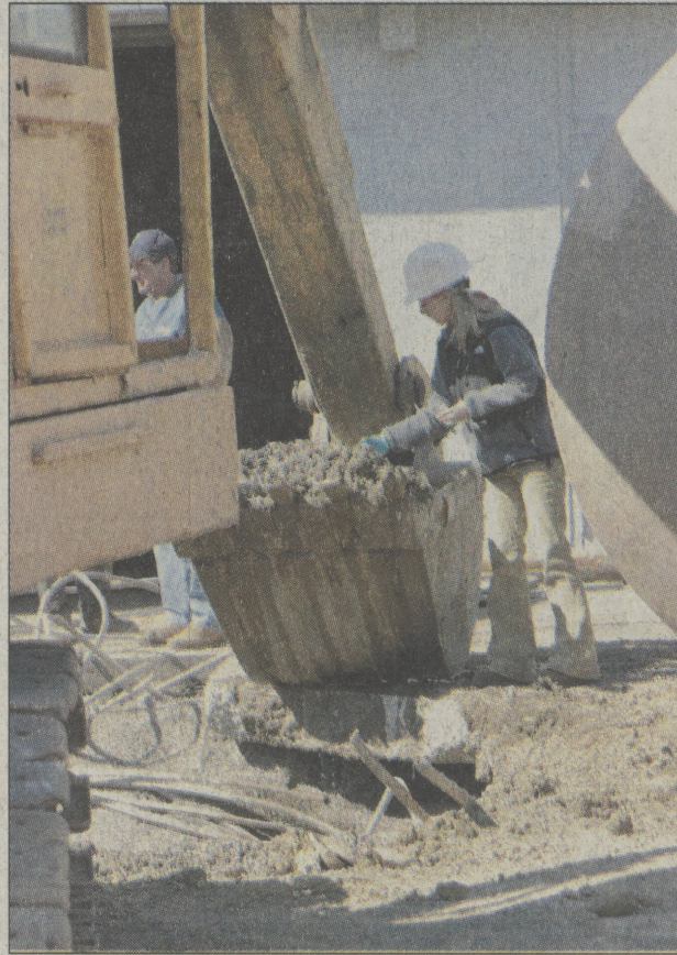
Jen Hindman from Aquaterra Technologies, a West Chester-based company hired by Sunoco, tested the ground and water as tanks were taken out of the closed gas station at the center of Dallas. The station is being removed to make way for improvements at the busy intersection, which will allow the developer of land in Dallas Township to proceed with a project there.
