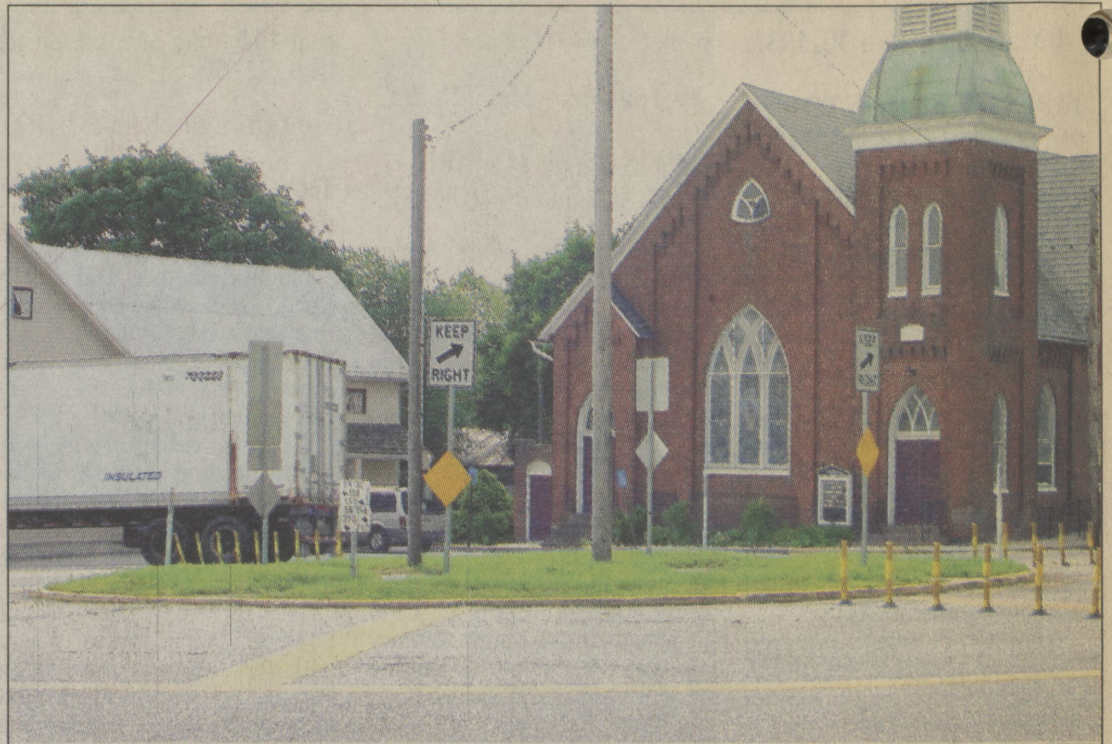
Abbottstown's roundabout is the smallest diameter PennDOT builds, yet it handles as much traffic as Memorial Highway through Dallas Borough.
