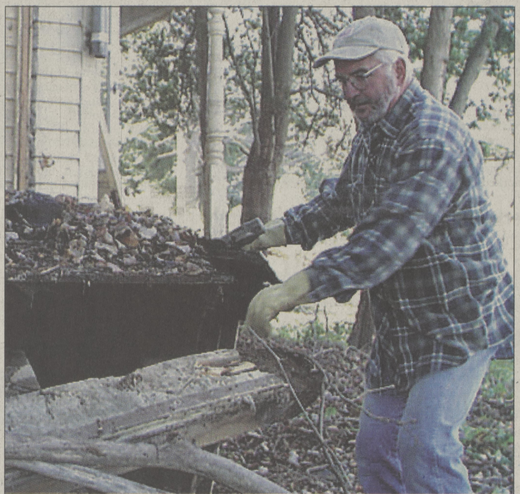
Joe Hudak helped take down the rotted back porch.
