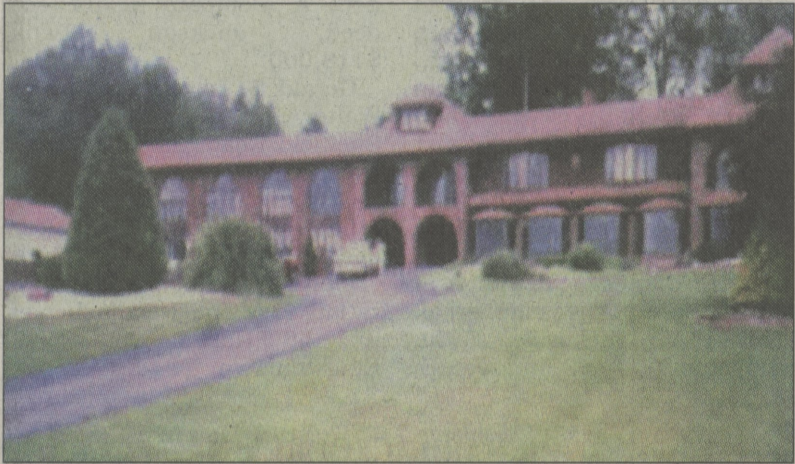
The Morrow mansion at 160 Lakeside Drive, Harveys Lake, as it appeared until last week, when it was demolished.
