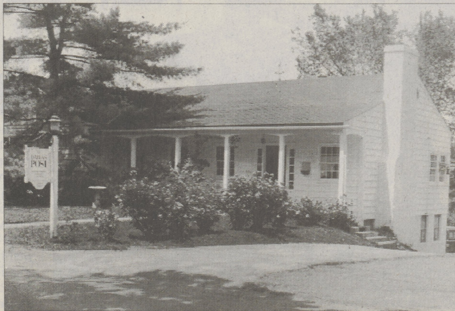
1930's to 1970's - Under Howard Risley's stewardship, The Dallas Post occupies an office on Lehman Ave.
