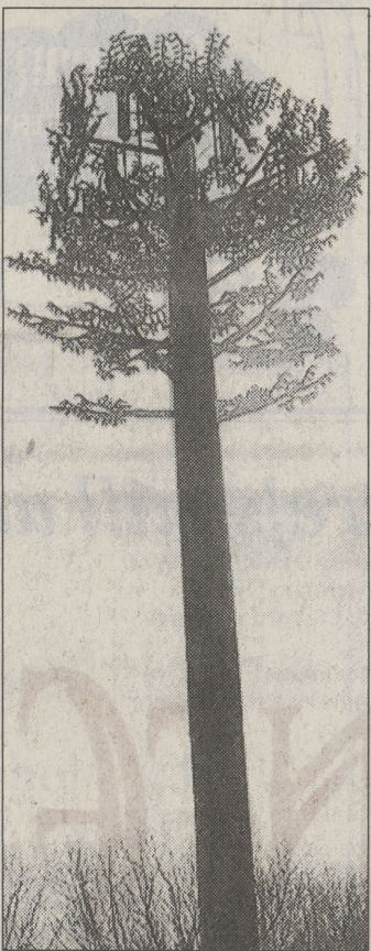
This is a cellular phone tower, dressed as a tree. Some communities require that towers be disguised.
