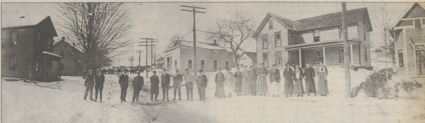
This photo shows the present Besteder home, right center, as it appeared when it was the office for Commonwealth Telephone. Most of the employees are identified. From left, Clarence Gay, Clarence Boston, unidentified, Walter Sickler, Ira Walters, Olin
