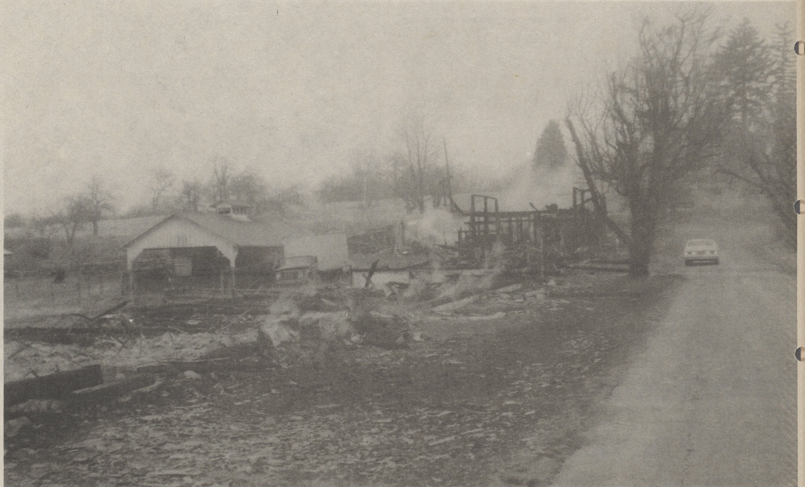
Two days after the fire, smoke still rose from the ruins of the Hayfield barns that burned Dec. 2.
