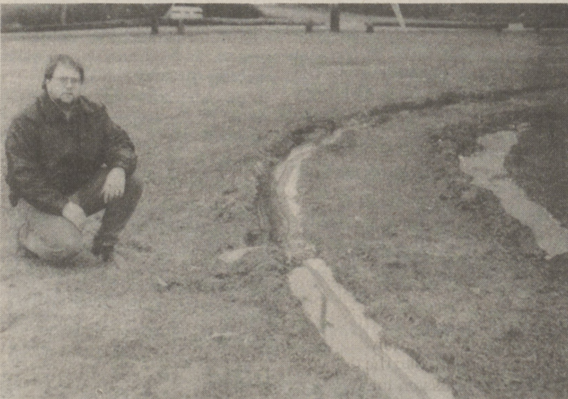
Mark Kraynak, supervisor of buildings and grounds at the Dallas School District, surveys the 12-inch deep ruts which the driver of a four-wheel-drive pickup truck left on the lawn of the high school last week.
